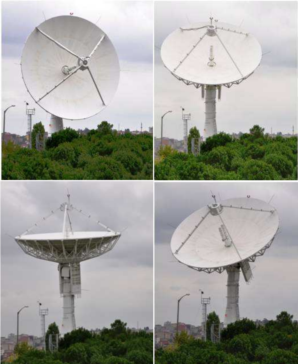
Figure 4: Motion of the 13 m diameter antenna
