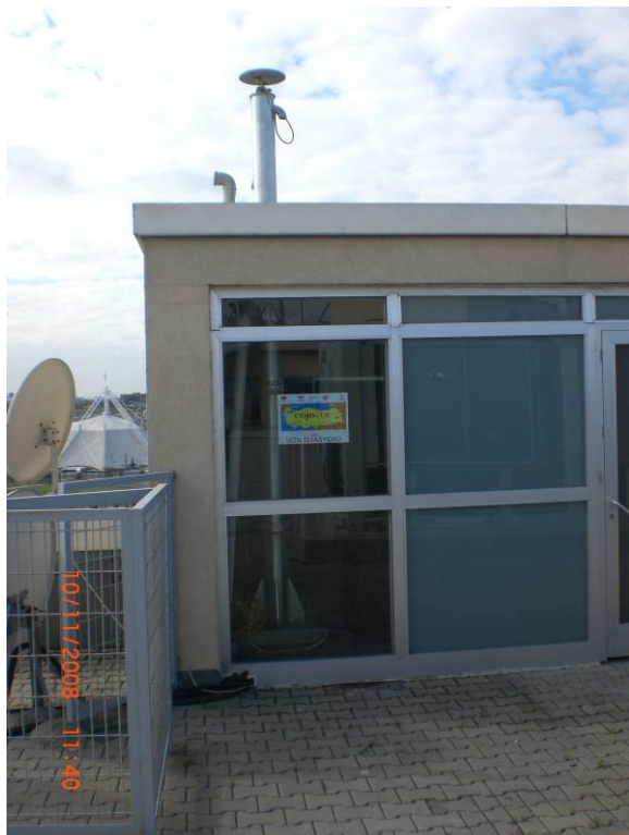
Figure 3. The CORS-ISTN station
